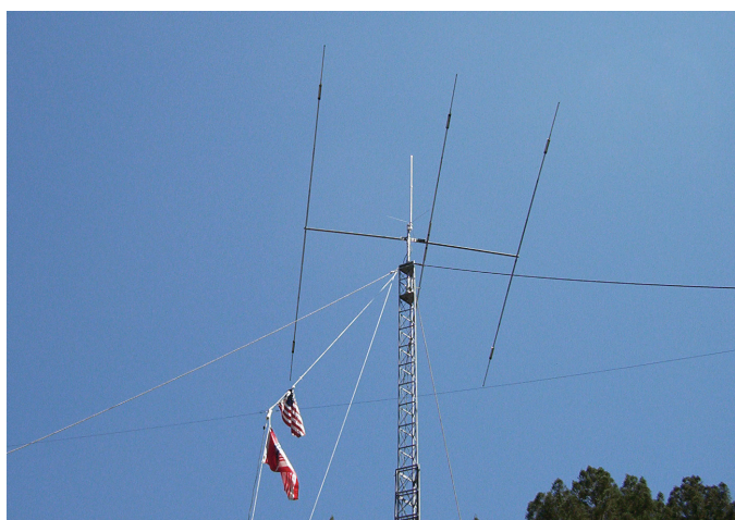
Antenna tower at the phone station... On the beam, it looks like we put the driven element closer to the director than the reflector—that explains the funny pattern we were getting.
